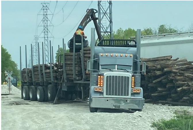
Figure 3: Boom truck loading ties for disposal
