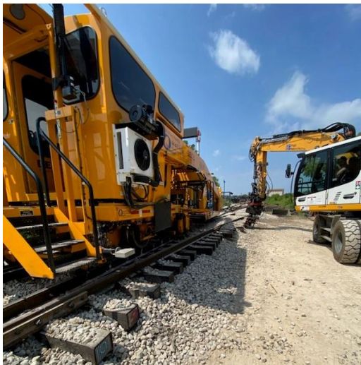
Figure 4: PNR Railworks Mark IV tamper
